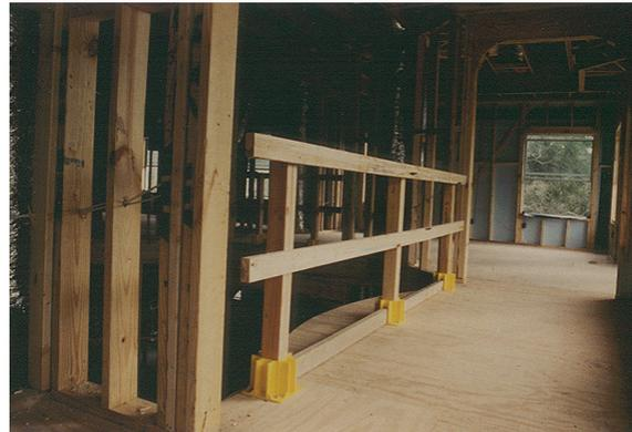
This Safety Boot Guardrail System (which includes toeboard slots), its construction and installation, meets OSHA regulations.
